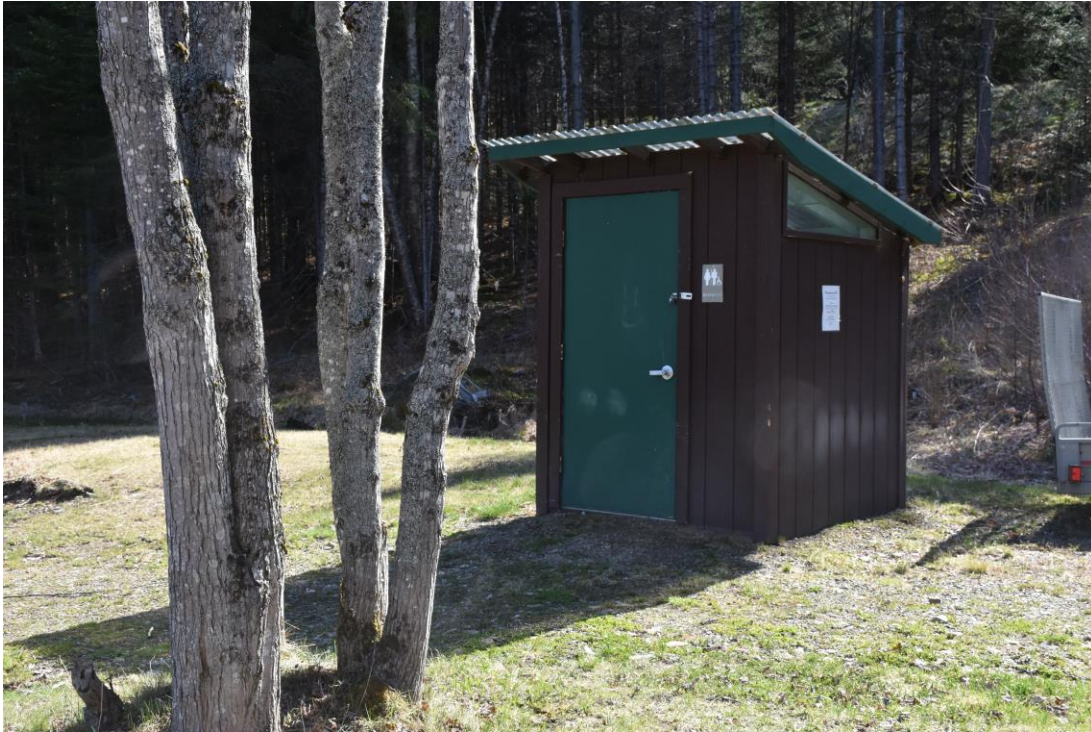
Photo 14) Temporary pit toilet ca. 2020 Reference (file name): PIC_2482
