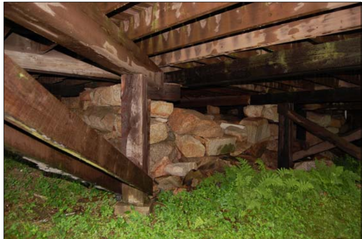
Photograph 5-1. Possible foundation stones from the Willey House Hotel under the current Restaurant Building, view northwest, Willey House Site, Crawford Notch State Park.
