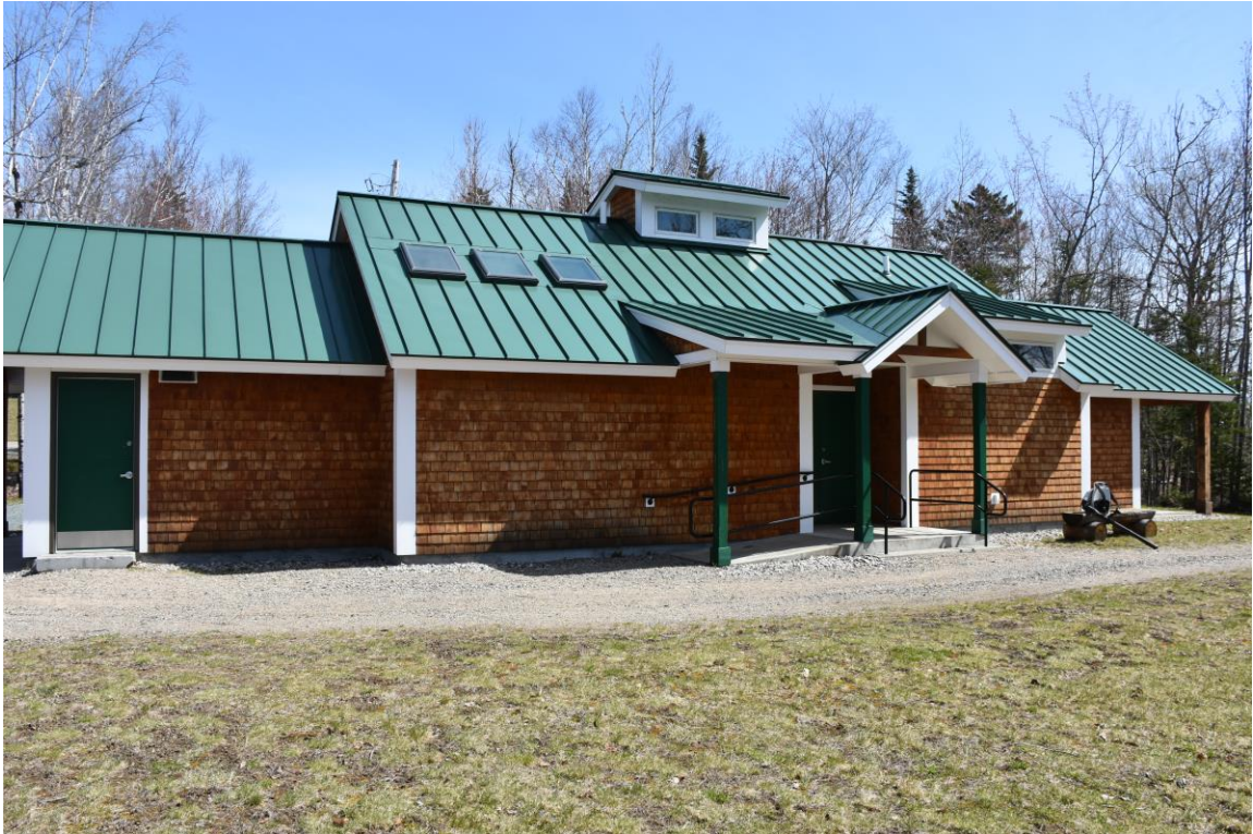
Photo 14) Bathhouse, built ca. 2016 Reference (file name): PIC_2608
