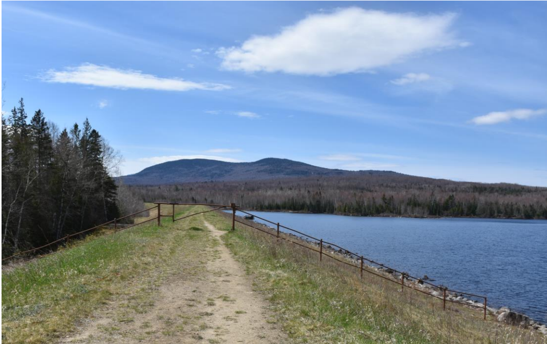
Photo 26) Dam fence and gate Reference (file name): PIC_2633
