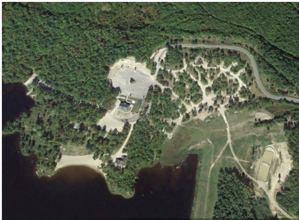
2013 satellite view showing new visitor center, event area and rebuilt campground (Google Earth)
