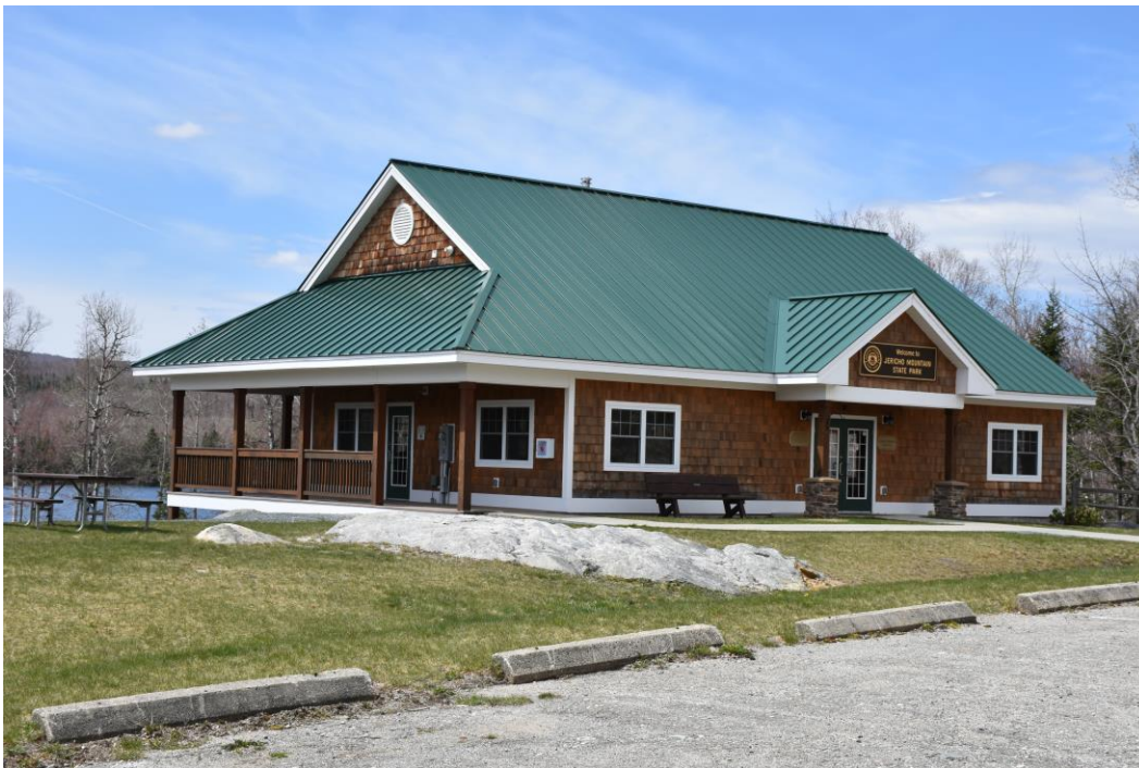
Photo 8) Robert A. Danderson Visitor Center built ca. 2011 Reference (file name): PIC_2664
