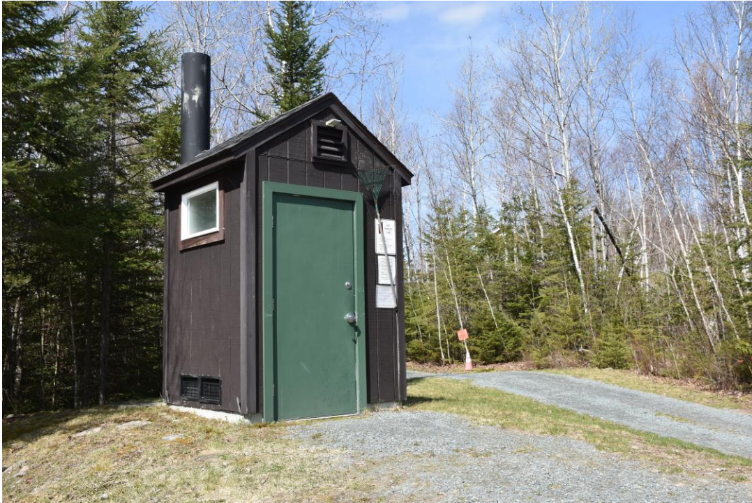
Photo 35) Pit toilet, ca. 2013 Reference (file name): PIC_2617
