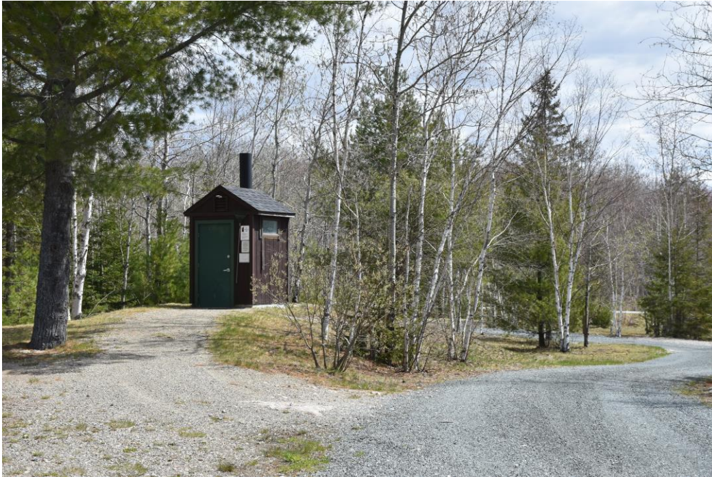
Photo 39) Pit toilet, ca. 2013 Reference (file name): PIC_2657
