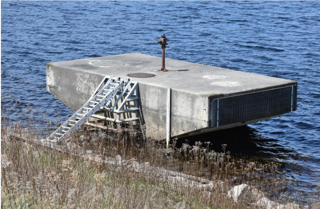
Photo 28) Dam drop inlet spillway gate Reference (file name): PIC_2640
