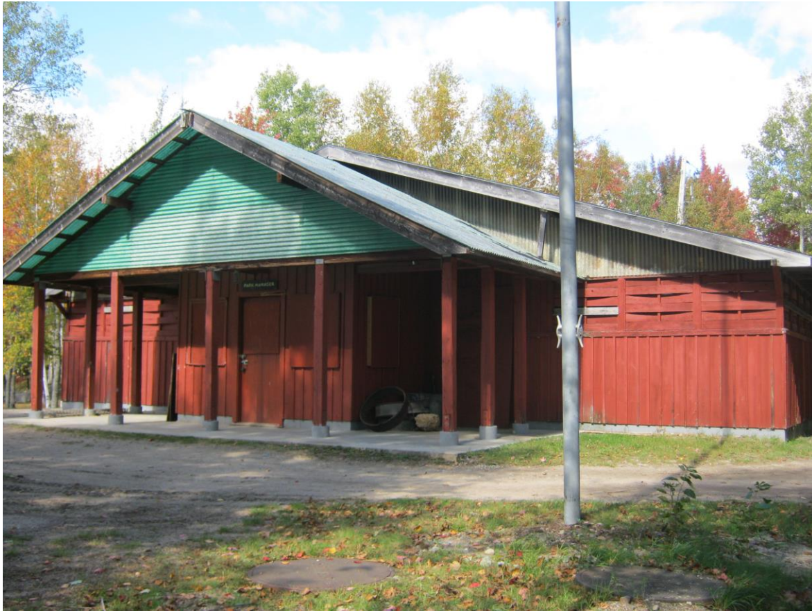
Old bathhouse built ca. 1975, replaced 2016 (NH Division of Parks and Recreation)
