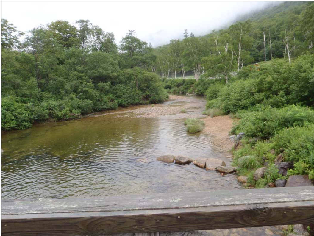
Photograph 3-2. General view of the Saco River from on top of the Willey House Dam, view southwest, Willey House Site, Crawford Notch State Park.
