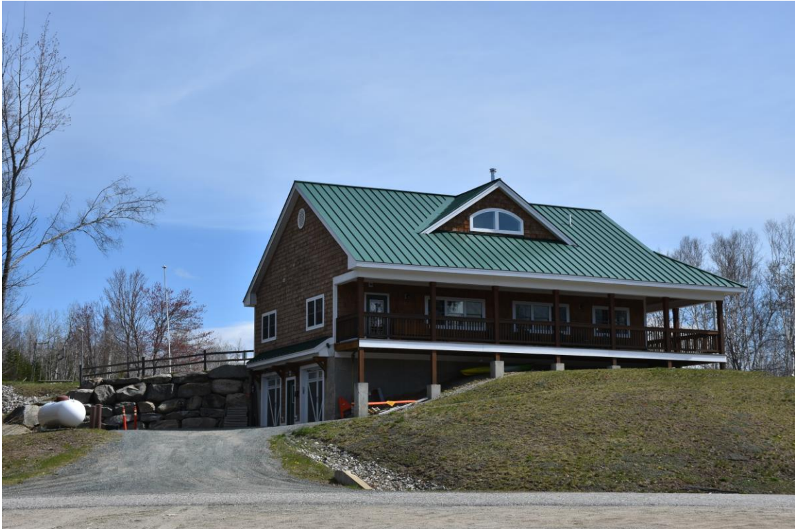
Photo 9) Visitor Center from beach parking lot Reference (file name): PIC_2579
