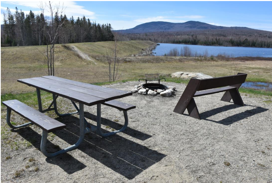
Photo 4) Dam from campground, showing emergency spillway area between
