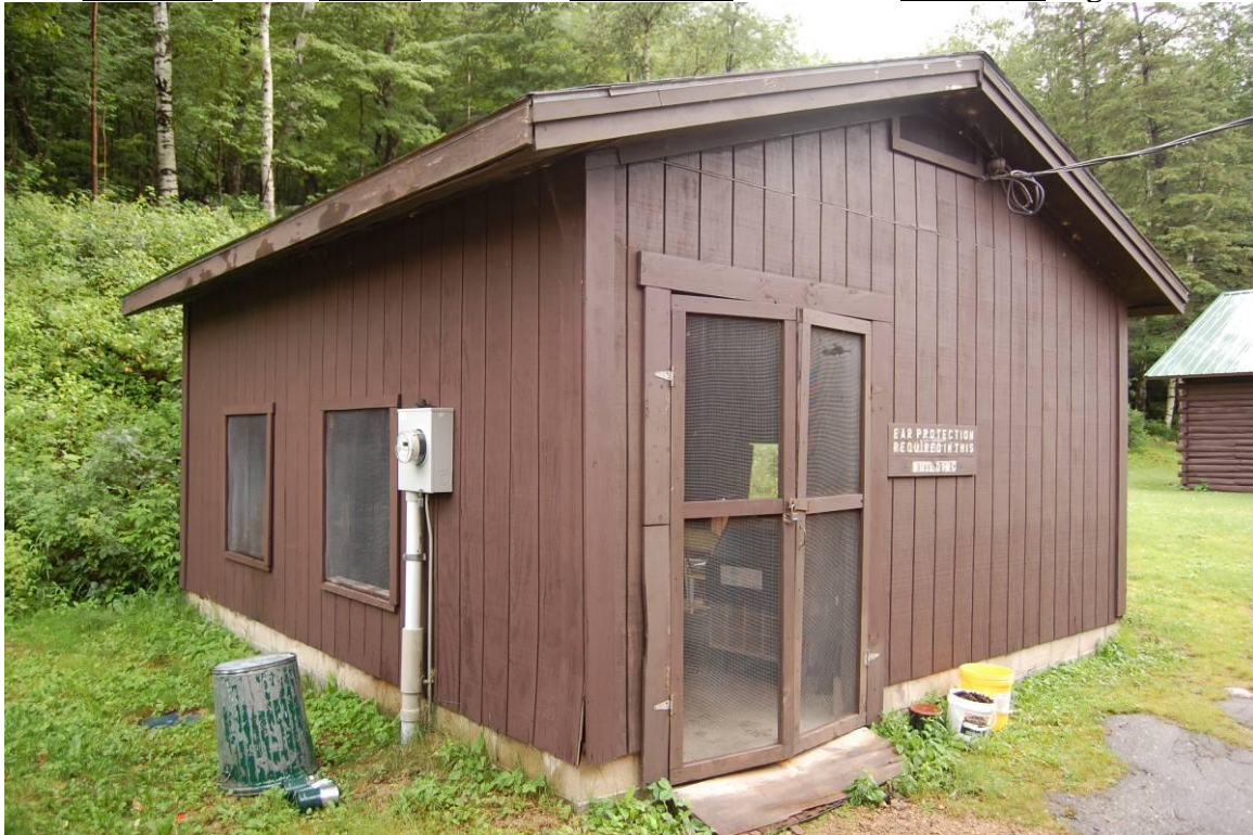
Photo 12 description: Generator House (CRW02, map no. 8)
