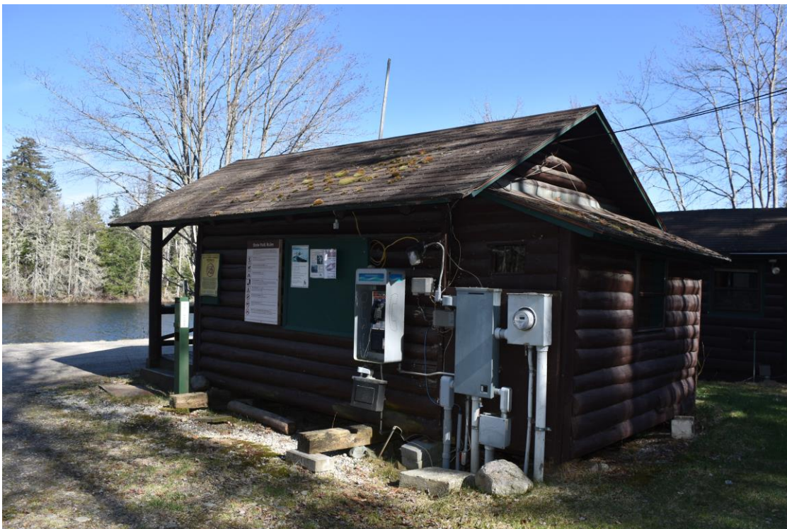
Photo 4) Office cabin north and rear elevations Reference (file name): PIC_2504
