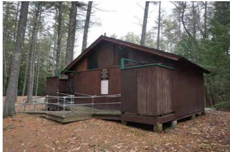
CAMPGROUND TOILET BUILDING, PAWTUCKAWAY STATE PARK
