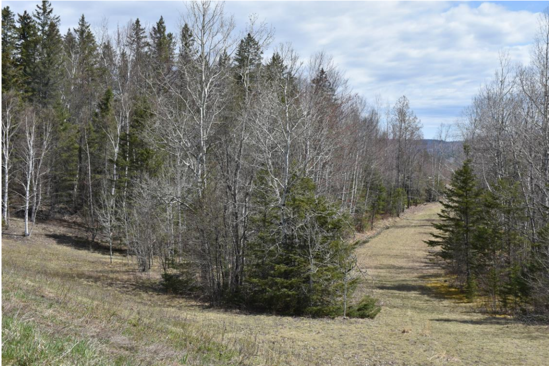
Photo 30) Former dam access road from top of dam Reference (file name): PIC_2650
