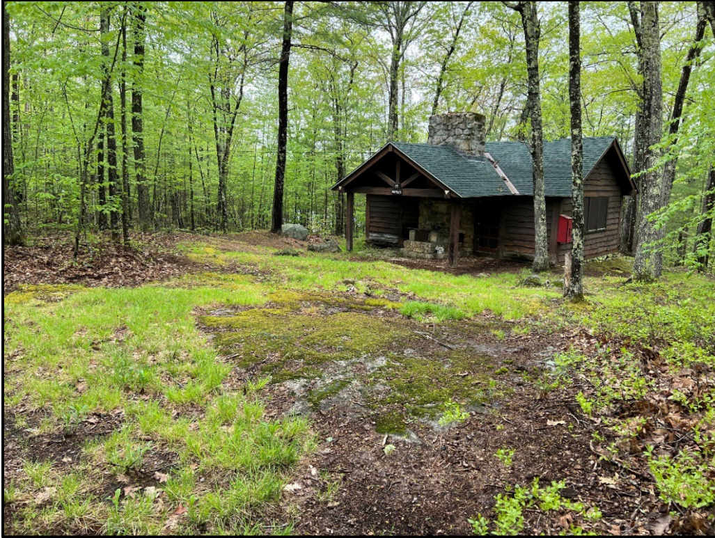
Plate 5. Exposed Ledge in “The Maples” Cabin Group, View West-Southwest
