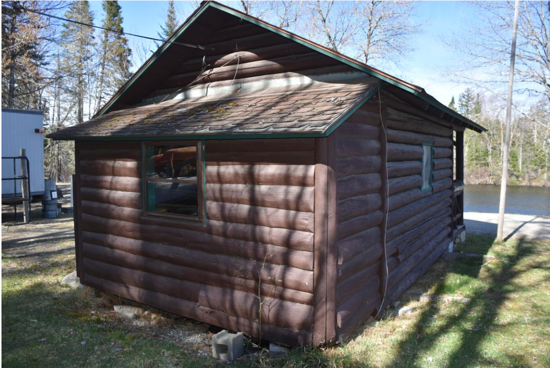
Photo 6) Office cabin rear elevation Reference (file name): PIC_2501
