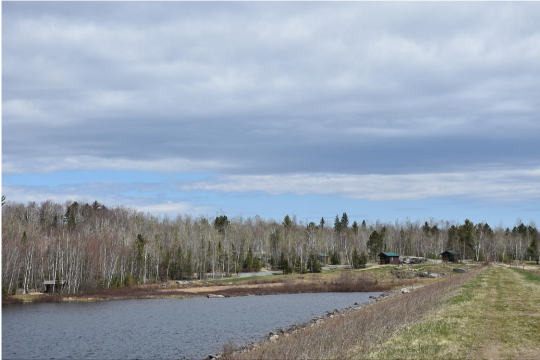
Photo 3) Campground shoreline viewed from top of dam
