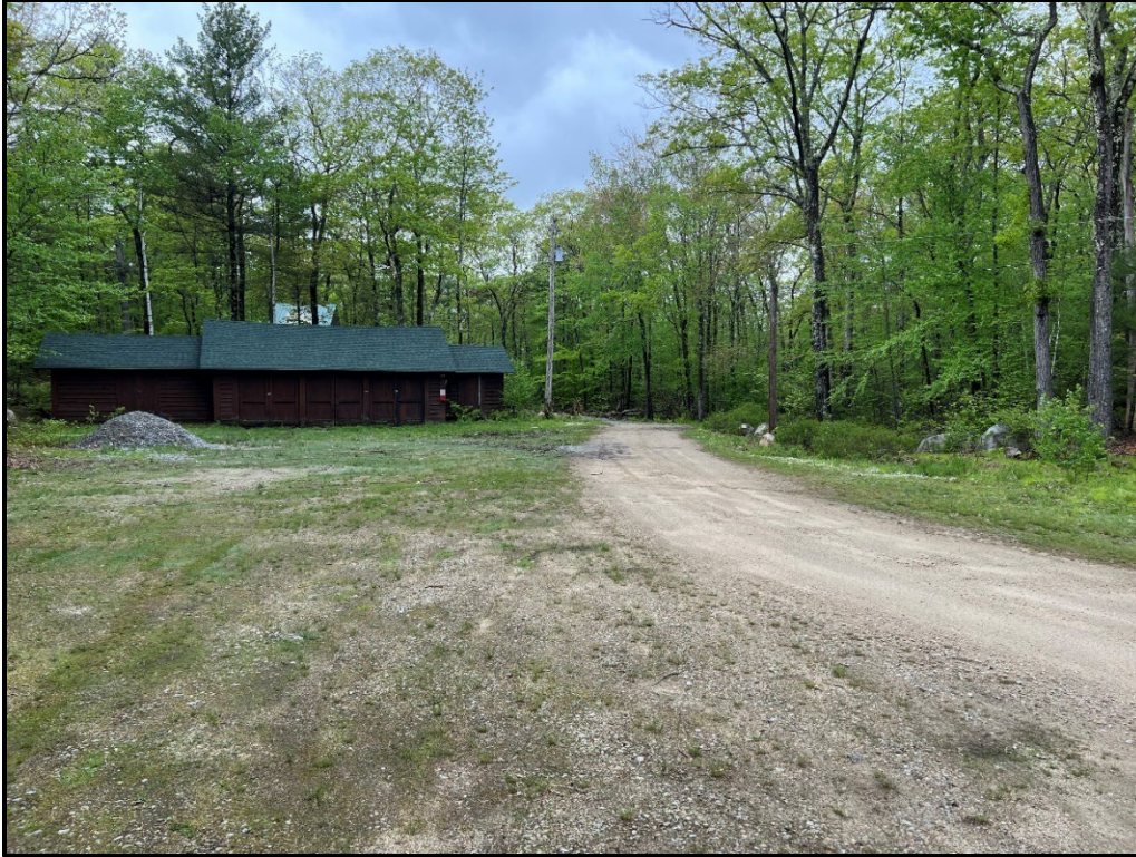
Plate 1. View Southwest of Proposed Parking Areas Showing Scraped, Rocky Terrain
